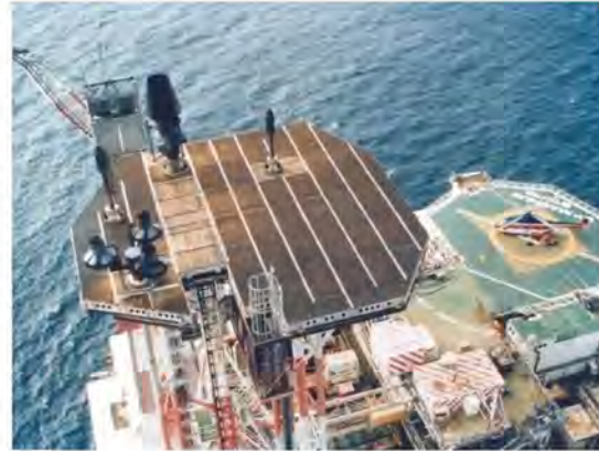
Darflare™ ‘chevron’ system installed on the BP Magnus Platform, UK North Sea
